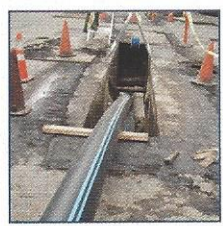
#1 in Trenchless Installations
